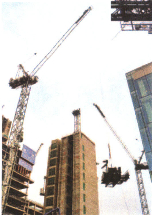
Left: At the New Street Square Building project an all new Potain MT225A was installed on the concrete core using a Potain MR220
