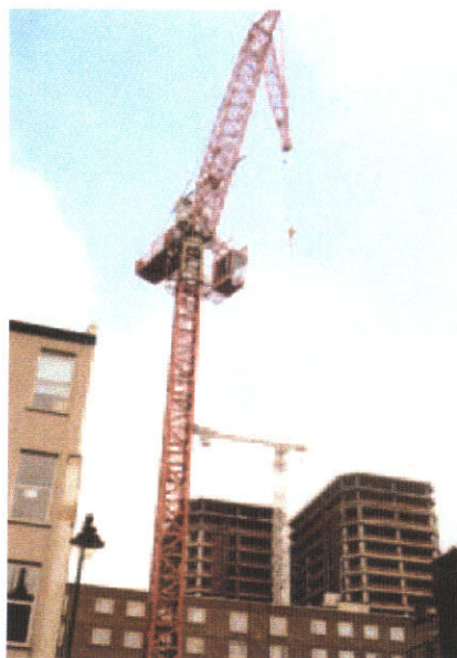
Left: At the New Street Square Building project an all new Potain MT225A was installed on the concrete core using a Potain MR220
