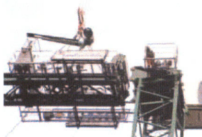
Left: At the New Street Square Building project an all new Potain MT225A was installed on the concrete core using a Potain MR220
