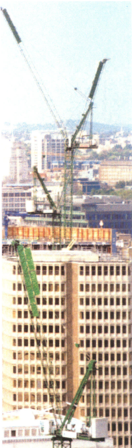
For a house building site at Luking Street, Kier Plant delivered this Liebherr 160 HC-L with 55 m jib. In the one fall operation 8 tonnes can be lifted to 25 m radius and 2 tonnes at 55 m radius
