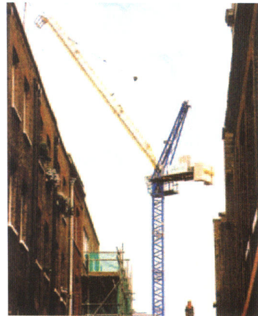
Clearly designed as a city luffing jib crane, this Jaso J80PA supplied by Falcon Crane Hire on a 1.18 x 1.18 m tower system is rigged in the backyard of a renovation project at Great Sutton Street. At 25.5 m radius capacity is 3.5 tonnes
