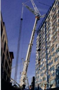
In position on one side of the confined site, the luffing jib of the Baldwins Crane Hire Liebherr LTM 11000D was used to reach right over the top of the new building
